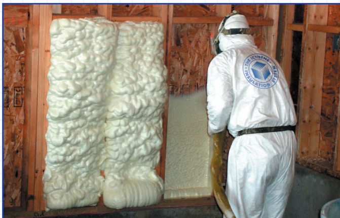
When sprayed in place, Icynene® forms a continuous blanket of soft foam that restricts air movement around electrical boxes and through other openings in the structure.
