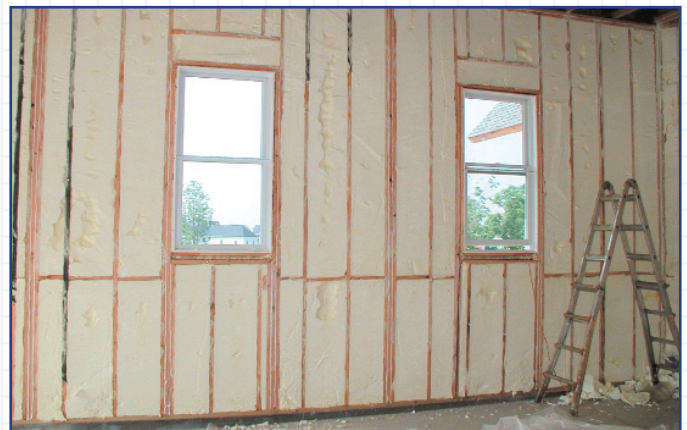
Insulating with Icynene® effectively minimizes the intrusion of outdoor allergens and pollutants, allowing the Knights to control the quality of their indoor air.
